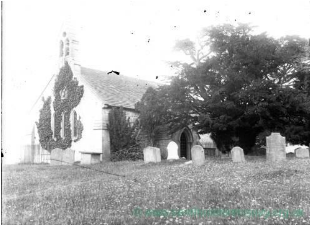
The Church before the bellcote was removed in 1961
